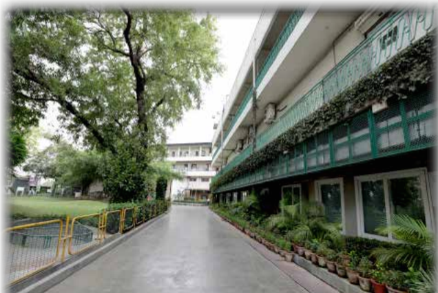
Administrative Block at Factory- MIL Hapur
